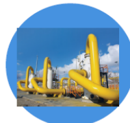
Gas Pipe Installation Area
