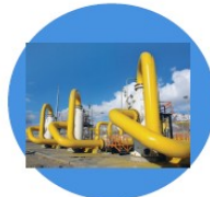
Gas Pipe Installation Area
