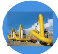
Gas Pipe Installation Area
